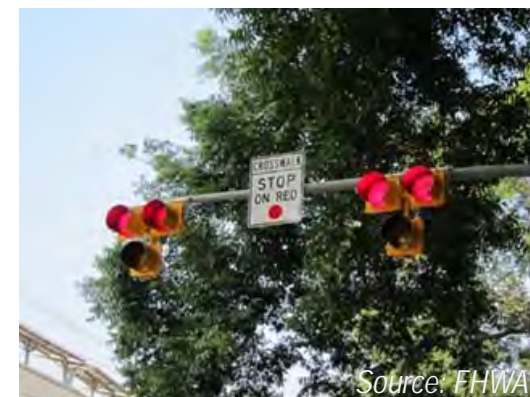
Pedestrian-actuated traffic signals (beacons)
